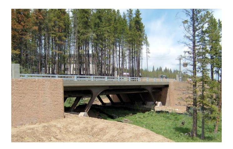
**Overview:** 3-Span, Steel Slant-Leg Girder &
